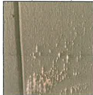
Sample #3: North Wall of Meeting Room on Wall panel above chair rail (Label 795)
