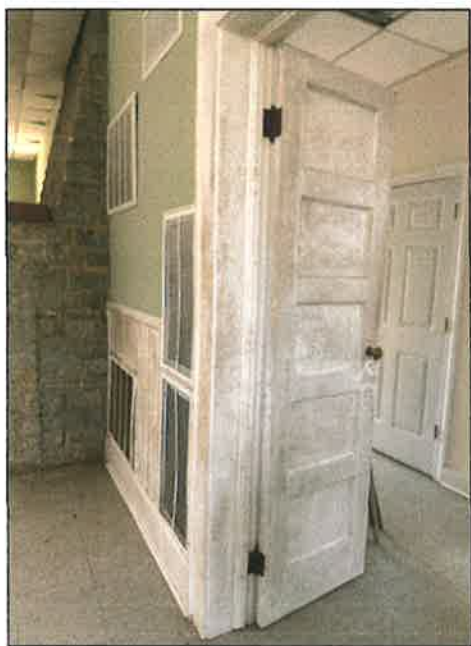
Entry into West Wing
