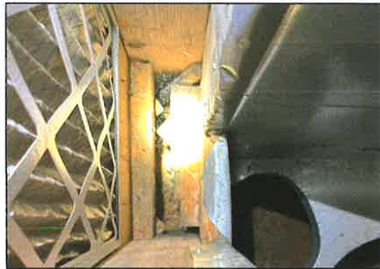
Note wall cavity between air filter and metal return plenum. Wall cavity communicates with crawl space
